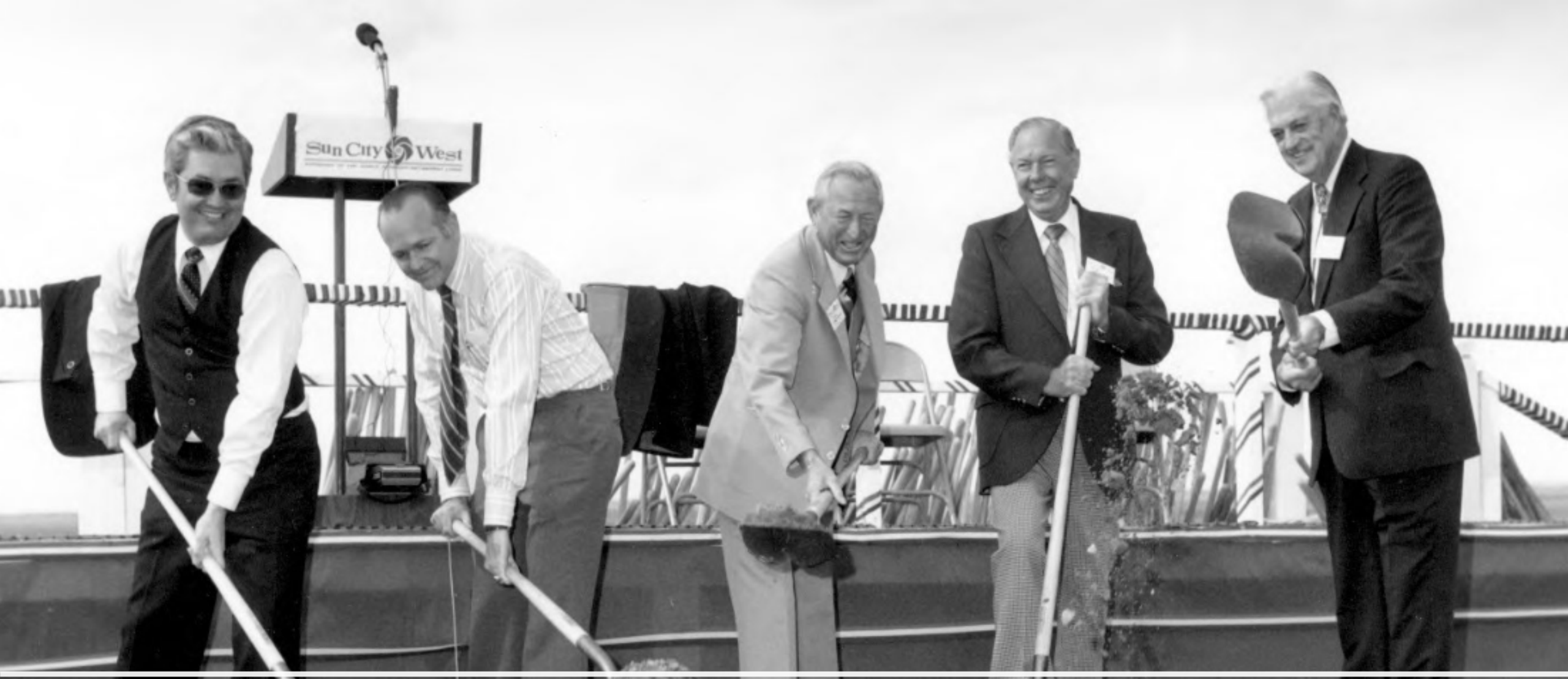
February 15, 1978, some 500 civic and business leaders attend the official ground-breaking for Sun City West
