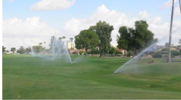
There are five sprinklers running in this fairway, all controlled by one valve. These sprinklers cover north- and south-facing slopes and high and low areas. Due to the system, all areas must receive the same amount of water. Ideally, they should controlled independently.
